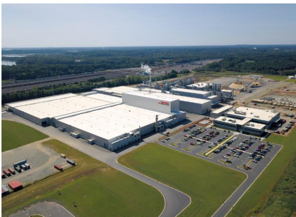
The 20th EGGER plant in Lexington, N.C. (USA) started operation in September 2020.
