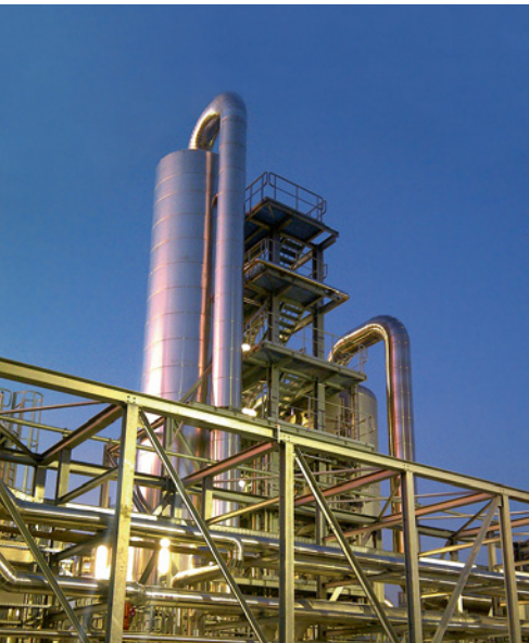
The Formox plant in Radauti (RO) turns methanol and water into formalin for resin production.
