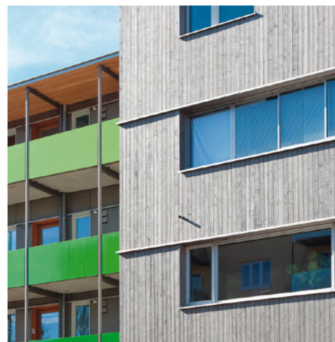
Self-carrying wood facade: the GWG Munich's award-winning rehabilitation of a 1950s building involved the addition of a prefabricated construction to the facade. It was fitted with windows and integrated building services.
