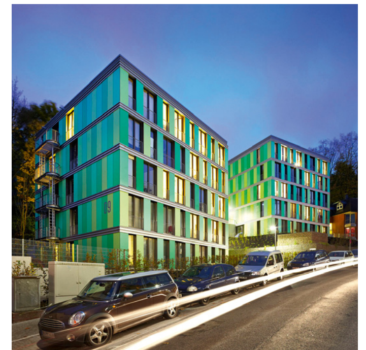
Reinforced concrete on the inside, timber on the outside: the windows and floor plans of the three new students' apartment buildings in Wuppertal can easily be adapted to new uses.
